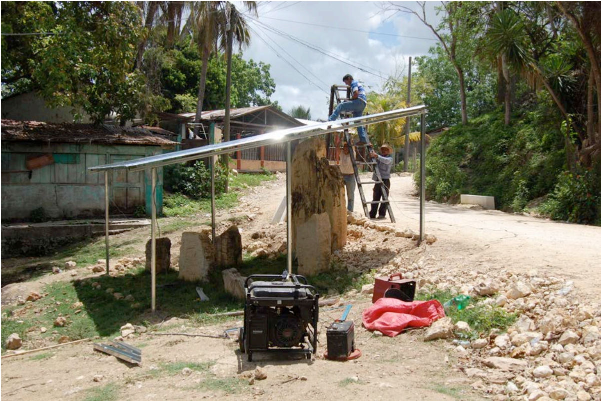
Completing the new roof.
